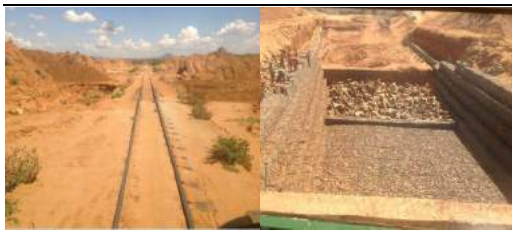
Figure 4-9 Heaps of Sediments Recovered from a Bridge at Existing MGR and Gabions being installed at Gode Gode
