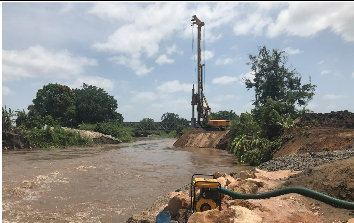
Figure 5.5 Example of Construction Activity at the Ruvu River
