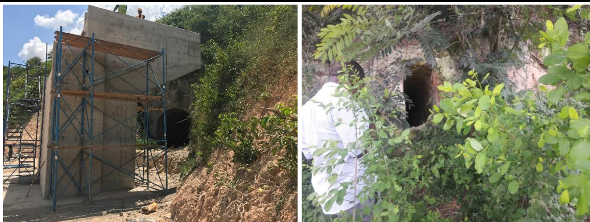
Figure 5.15 Old German Colonial Tunnel that needs to be destroyed (left) and an Old Mine Shaft (right) that was likely used by large numbers of Bats
